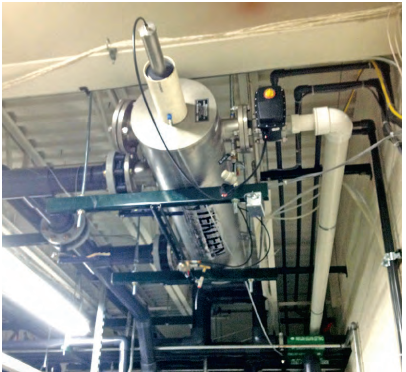
Tekleen filters installed at the Hoffer Plastics Corporation facility in South Elgin, IL
