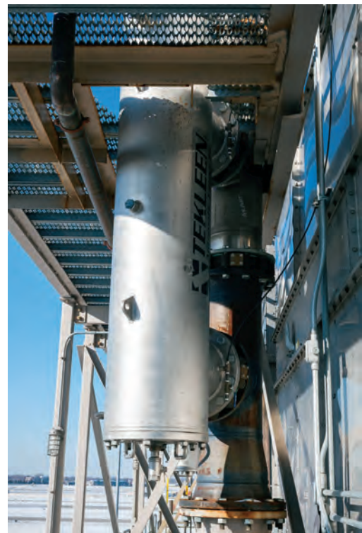
Close view of the Tekleen filter, vertical installation.
